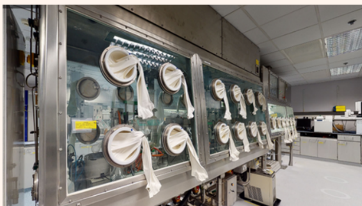
ADC payload facility in Ireland
